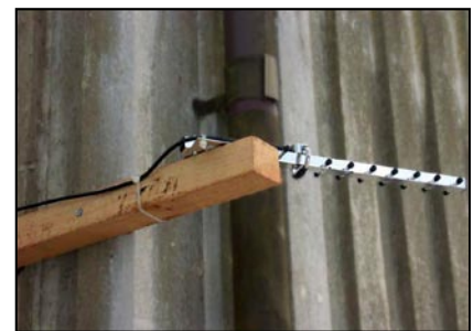
Example of how the A300 antenna should be placed
